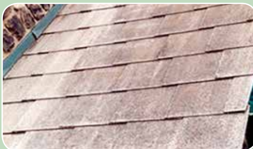
Asbestos cement shingles
