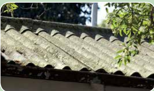
Asbestos cement corrugated roofing
