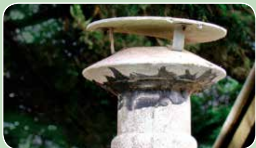
Asbestos cement flue and cowl
