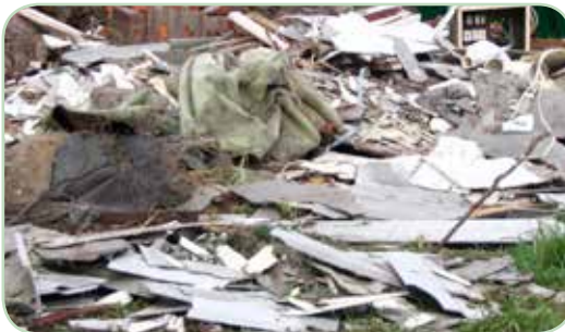
Broken asbestos cement materials from a demolition
