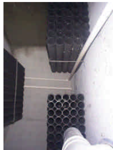
An example of fixed media looking down into an AWTS.
