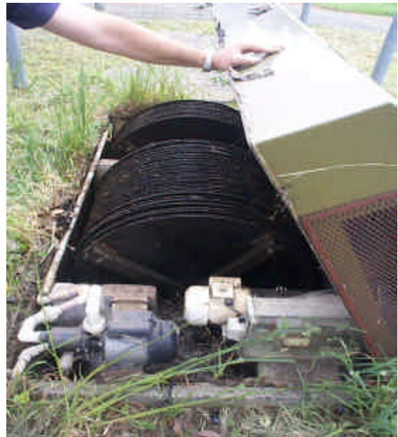
An example of a biological rotating disc system.
