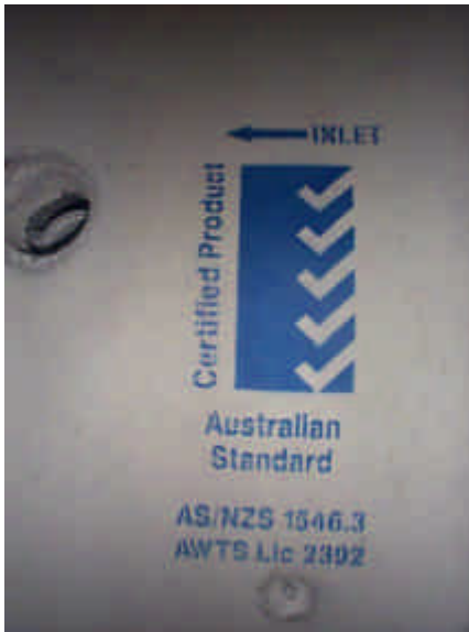
A photo of the required Australian Standards Markings for an AWTS.
