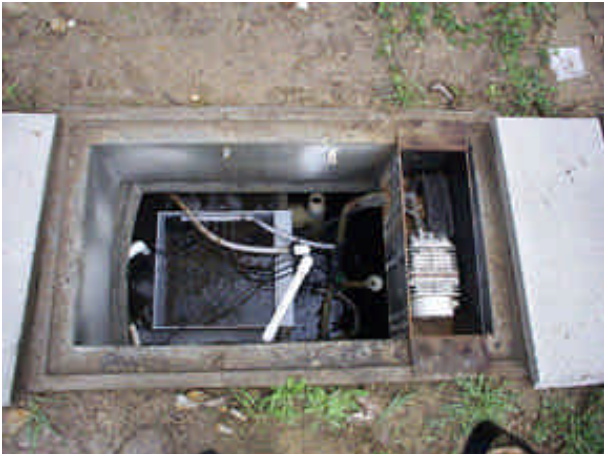
A view of an AWTS after installation showing some internal components.
