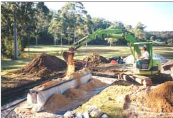
Figure 8.6 Backfilling with amended soil
