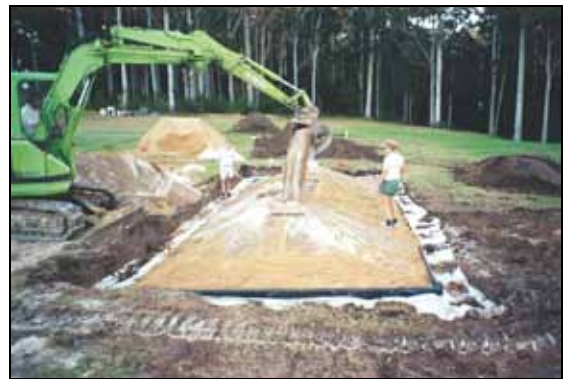
Figure 8.7 Final shaping of cell mound
