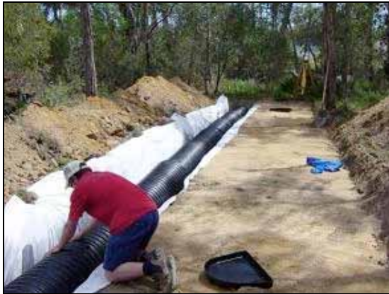
Figure 10.14 and 10.15 Laying the liner in the trench and then the geotextile fabric as the 'wick' across the pan
