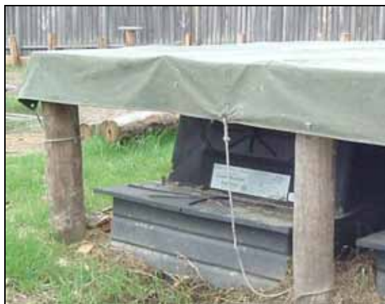
Figure 6.3 The installed composting unit, before installation of bathroom and steps
