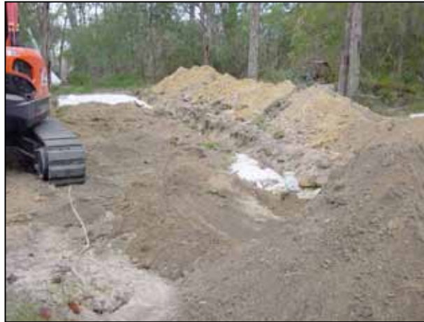
Figure 10.18 Backfilling and the inspection ports
