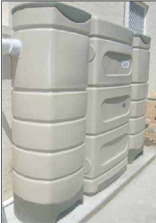
Figure 7.1 Example of an Oasis GT600 Greywater Treatment System (Nubian Water Systems, 2009)
