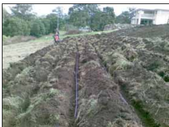
Figure 13.1 A subsurface irrigation system under construction (Smart Sewage Solutions)
