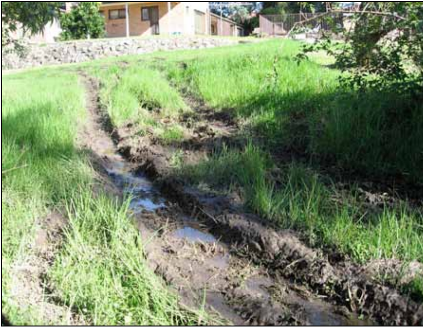
Figure 10.6 A failing trench due to vehicular activity
