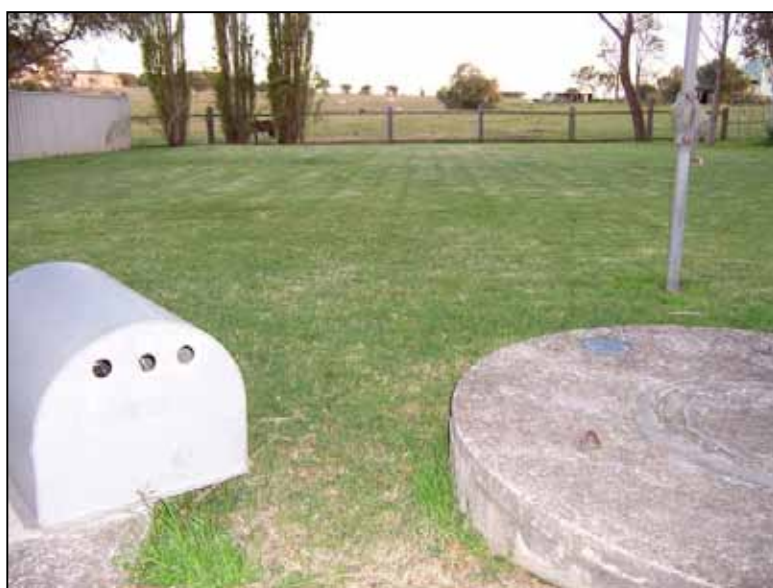
Figure 11.1 An evapotranspiration absorption bed
