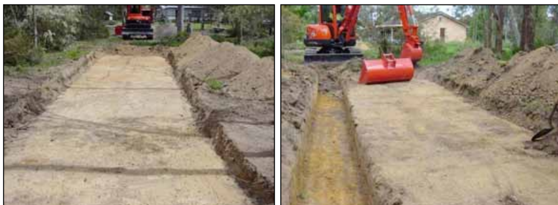
Figure 10.12 and 10.13 Excavation of the bed of the "Wick" trench
