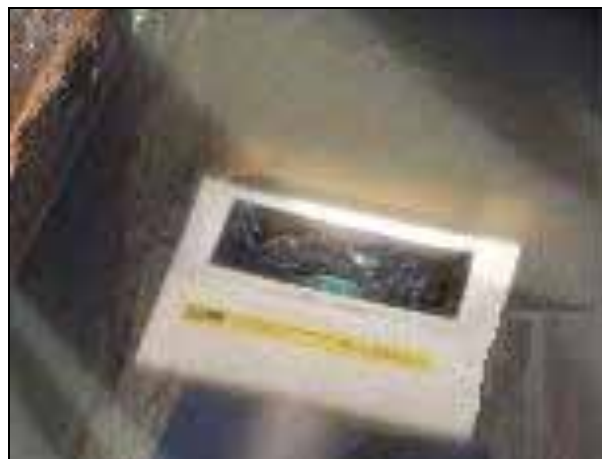
Figure 14.8 The dosing chamber continues to empty down to the top of the Flout ® (Figures 14.4 to 14.8 Rissy Plastics LLC)
