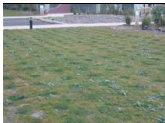
Figure 13.2 An installed subsurface irrigation system (Whitehead & Associates)
