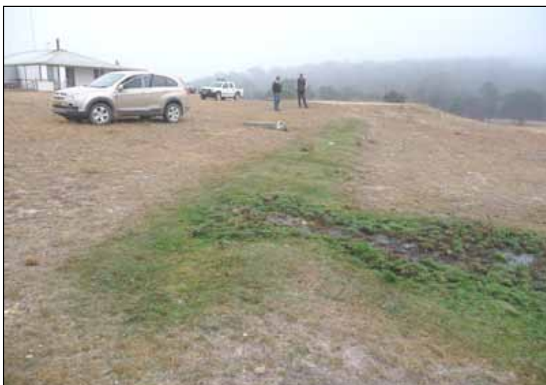
Figure 10.9 Failing trench
