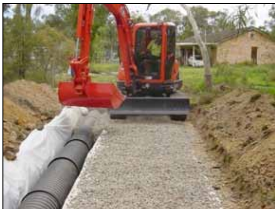
Figure 10.16 Backfilling gravel layer
