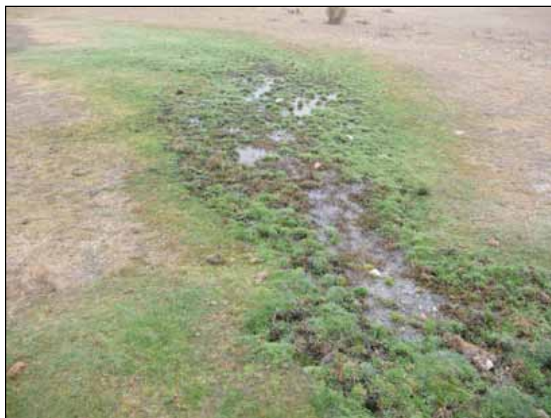
Figure 10.10 Failing trench
