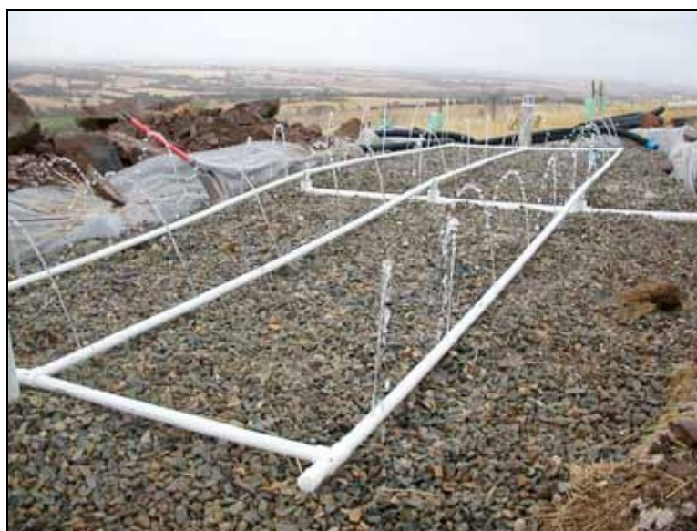
Figure 11.2 Pressure testing the distribution laterals for even distribution of effluent ( www.inwater.com.au )
