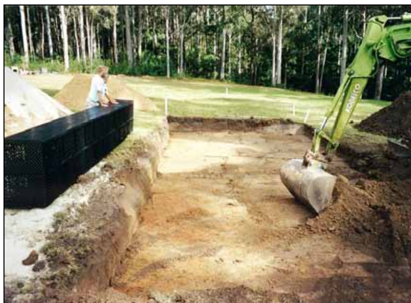
Figure 8.3 Excavation/preparation of base of mound (Figures 8.3-8.7 Ecomax, 2001)
