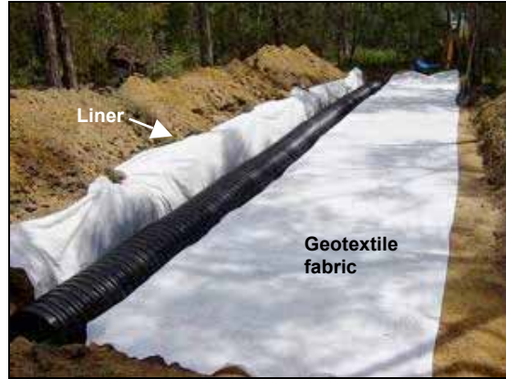
Figure 10.14 and 10.15 Laying the liner in the trench and then the geotextile fabric as the 'wick' across the pan
