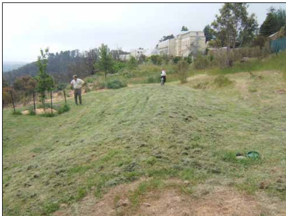
Figure 8.8 Finished amended soil mound
