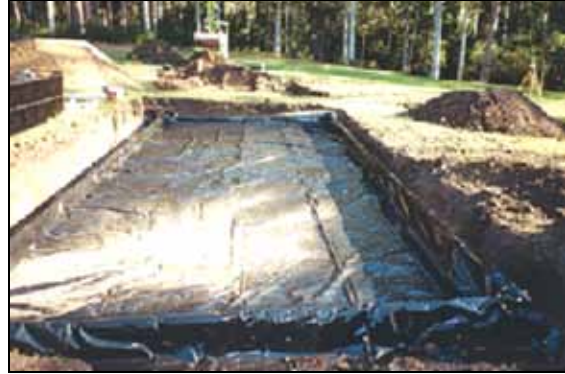
Figure 8.5 Lining with an impervious liner
