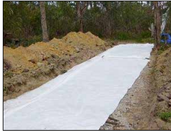
Figure 10.17 Adding the second geotextile fabric layer
