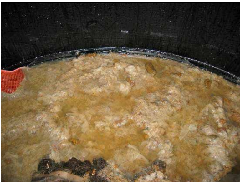
Figure 5.9 A flooded system due to pump failure
