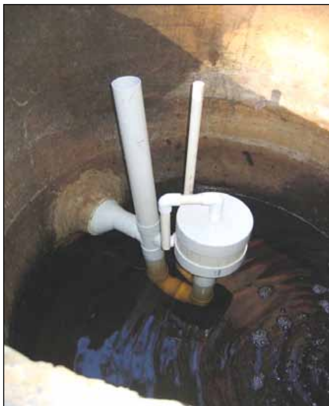
Figure 14.2 Dosing siphon in dosing chamber (Inwater)
