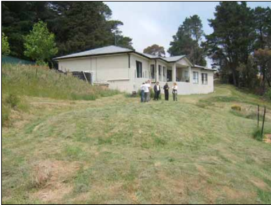
Figure 8.9 Amended soil mound constructed on sloping site
