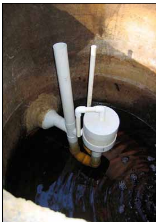
Figure 10.3 Dosing siphon (Inwater, 2010)
