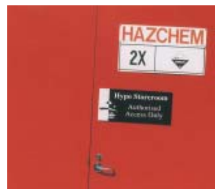
Figure 2 Hazchem signage for packaged dangerous goods
