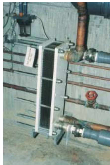
Figure 39 Gas fired direct pool water heater
