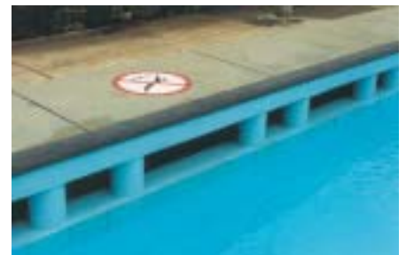
Figure 26 Overflow channel on an older outdoor pool
