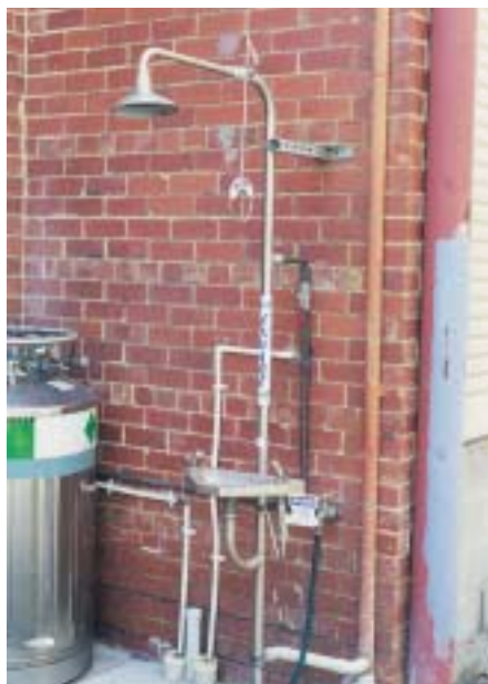
Safety Showers and eyewash facilities should be located immediately adjacent to the hazardous area, but not within the hazard.
